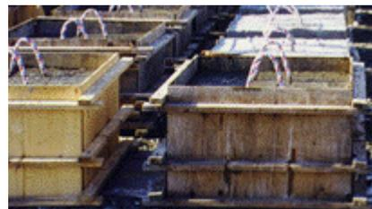
Figure 5 Square concrete block anchor
