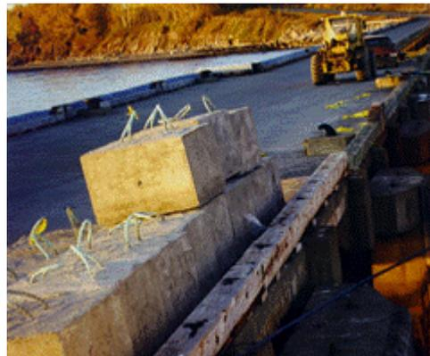
Figure 32 Anchor blocks loaded on dock
