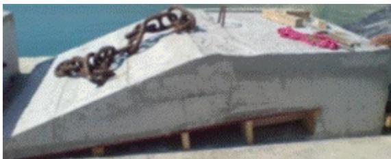
Figure 4 Wedge-shaped concrete block anchor
