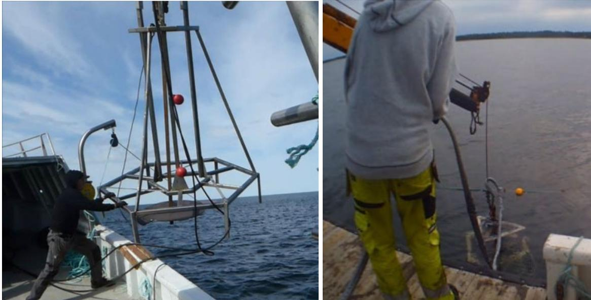
Figure 5. Left: Setting of the 20 helix side-anchors in 2016. It was hard to maneuverer the swinging drill-rig from a classic round-bottomed fishing boat. The original big plates shown in the picture were soon exchanged to smaller plates that could penetrate the sand-bottom. Right: Setting of 27 vertical anchors in 2017. This job was done with part of the rail removed, a new wooden deck, and perfect weather conditions.
